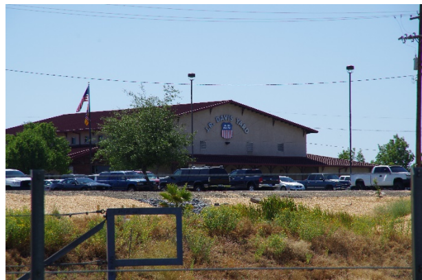
Photo 2-5: UP Railroad Yard.
