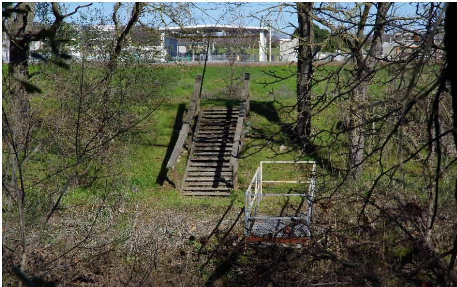
Photo 2-1: View of Roseville WWTP from Corp Yard.
