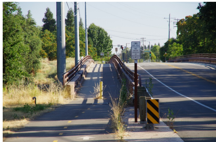
Photo 1-2: Existing multi-use path along Cook Riolo Road, looking north.
